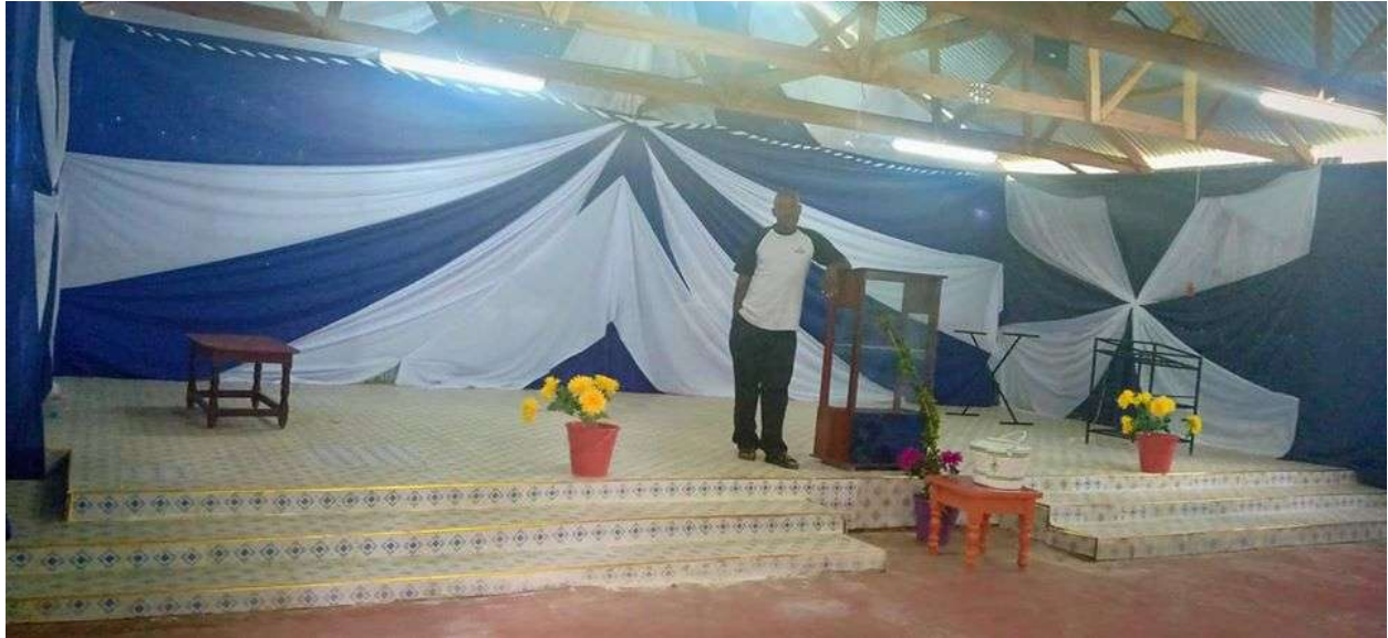
This is the tiled platform, that was just finished.
